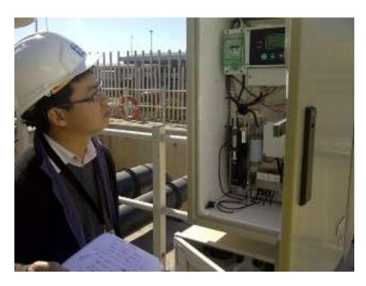
the transmission either immediately prior to the addition or after the addition of the first non-complex forming reagent. The term process photometer is preferred as the unit may be used for the measurement of low levels of chloride and sulphate by the measurement of the resulting turbidity formed on formation of the silver chloride or barium sulphate.
