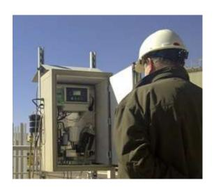
A simple external sample system may be required for the analysis of dirty wastewater process streams. The analysis of the water in aeration tanks, where sampling is made using a grinding pump, requires a small cyclone filter to remove the larger solid particles and provide a relatively clean (with only fines present) sample stream. The INSTRAN has a Turbo-Wash sequence in which any settled solids in the bottom of the reaction vessel are "thrown out" by the rapidly spinning stir bar.
